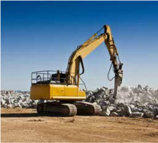
Machinery operated from a closed cabin
