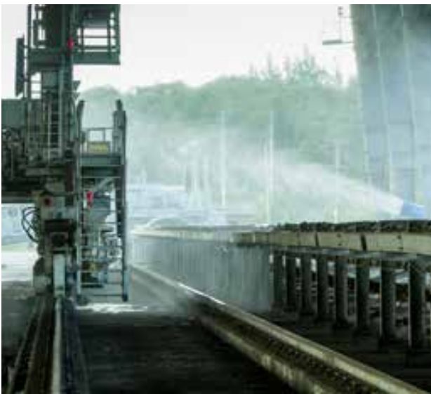
Conveyor wetting system
